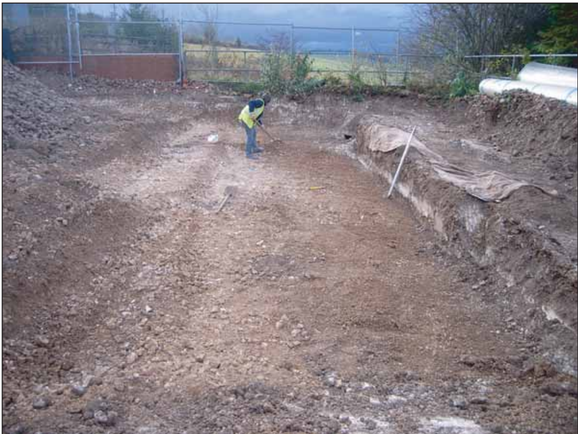
Plate 2: Area 2 viewed from the north-north-east
