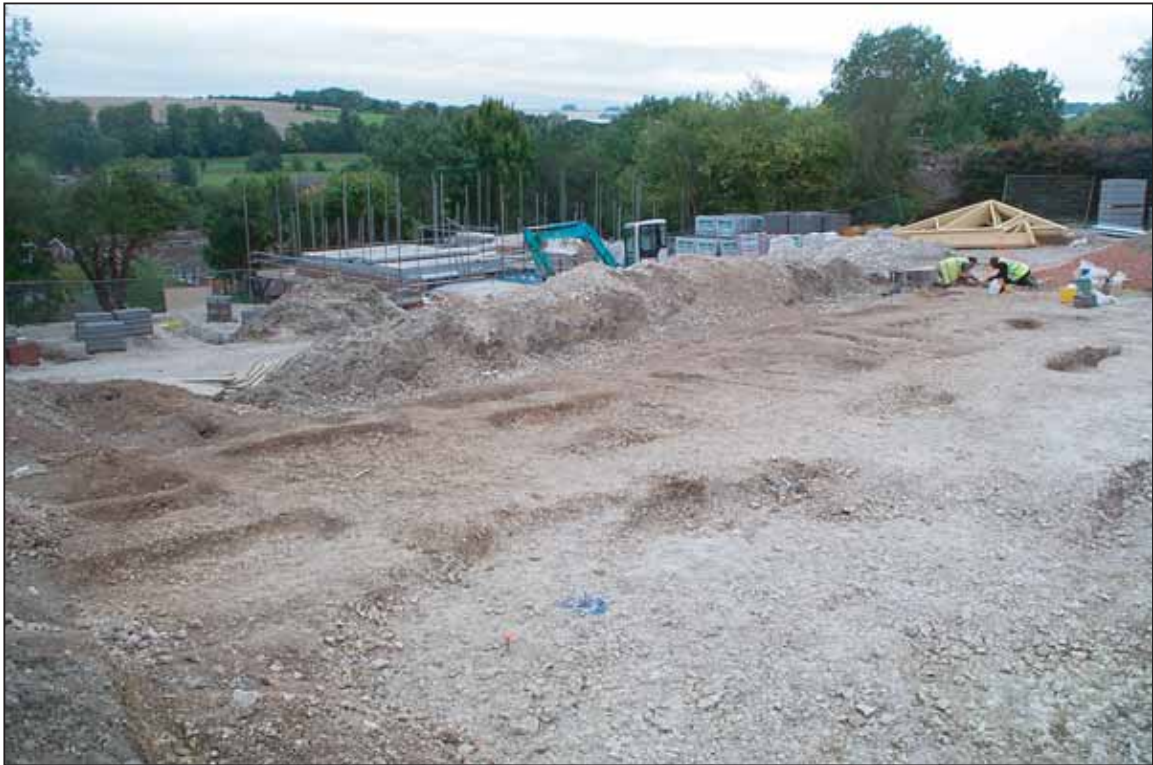
Plate 1: Area 1 viewed from the south-east
