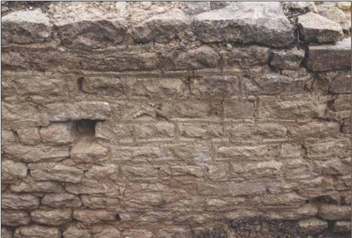
Plate 6. Caldarium (hot room); north wall (west end) showing struck pointing (no scale; view from south)
