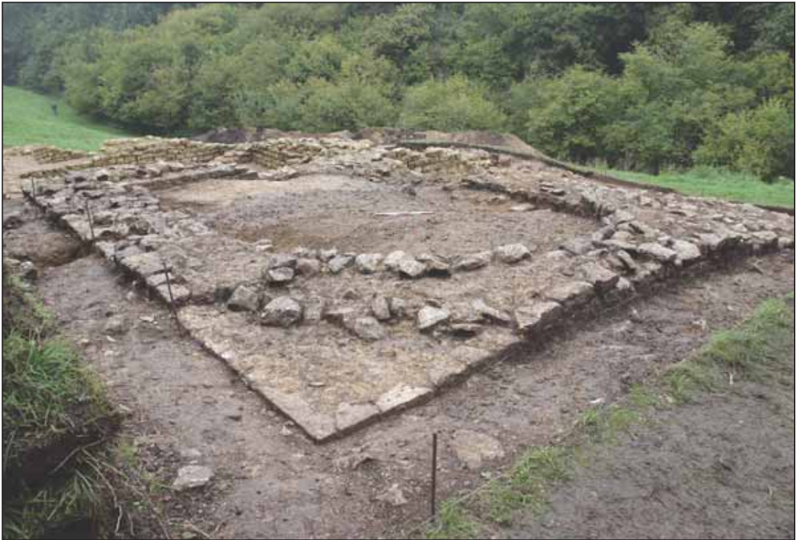
Plate 5. Caldarium (hot room); apsidal / square south end exposed (scale = 0.5m; view from south-west)
