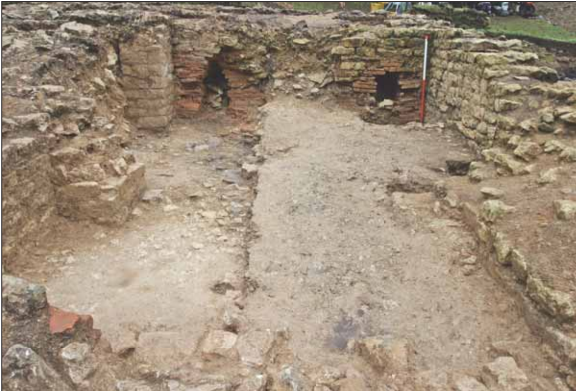
Plate 4. Tepidarium (warm room); annexe in foreground, flues between hot room and warm room in background (scale = 1m; view from east)
