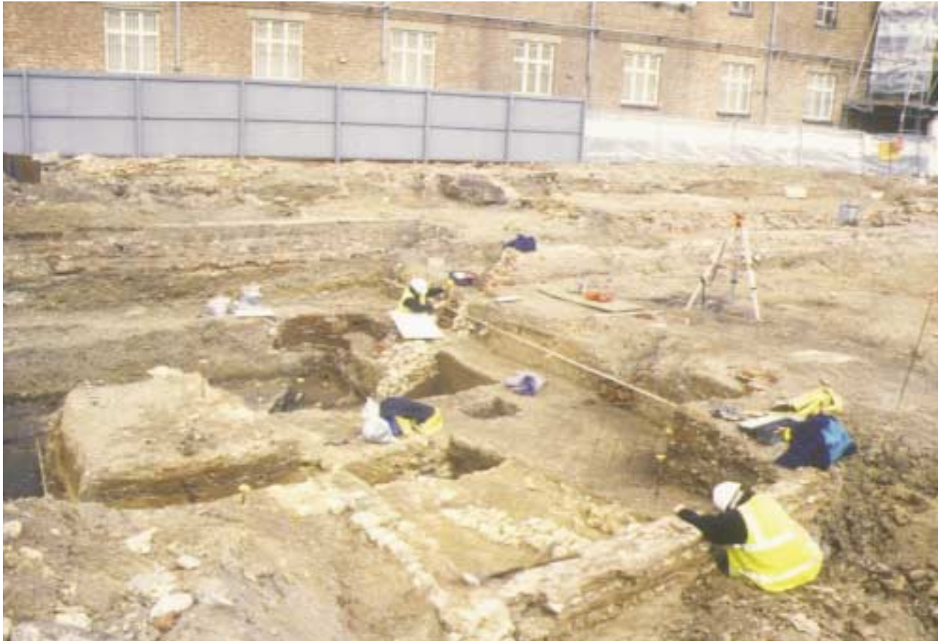
Figure 38: Excavating the foundations of a series of medieval buildings constructed over the edge of the infilled channel.
