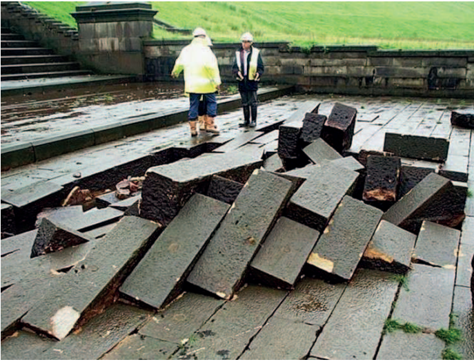
Severe damage to spillway caused by minor flood in 2002
