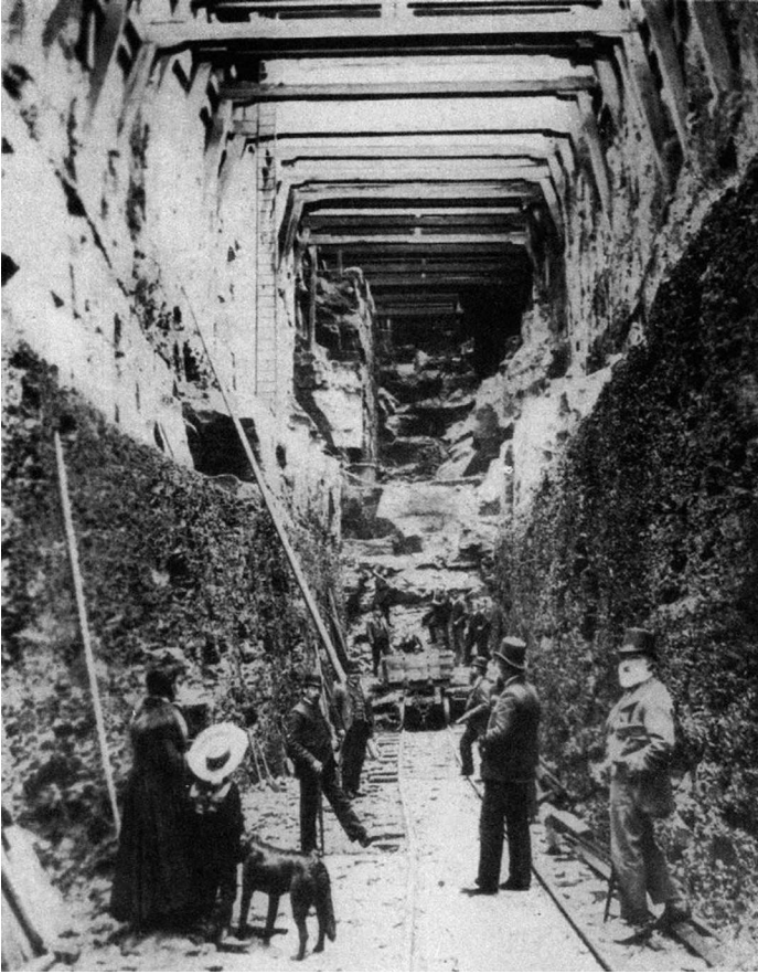
The puddle trench at Butterley Dam under construction
