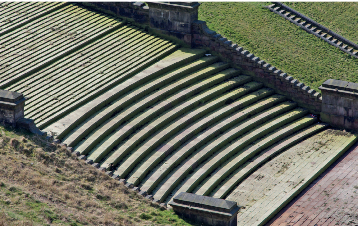
The original masonry of the spillway
