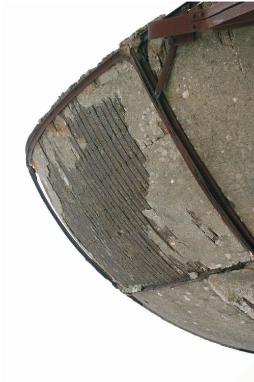
View of internal iron mesh of Sound Mirror from W
