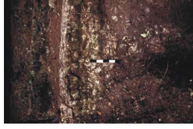
Plate 10: View of Trench 4 showing probably Victorian culvert wall. Looking east, 0.5m scale
