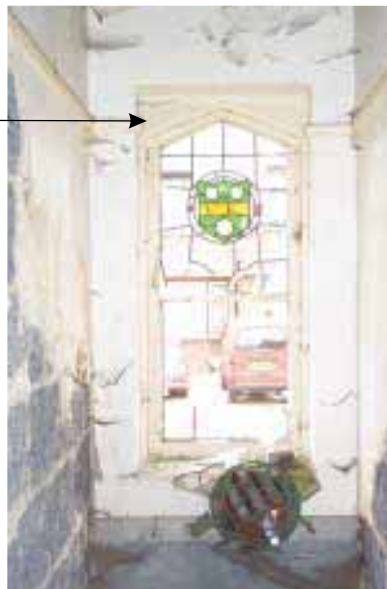
Plate 2: Stairwell window detail
