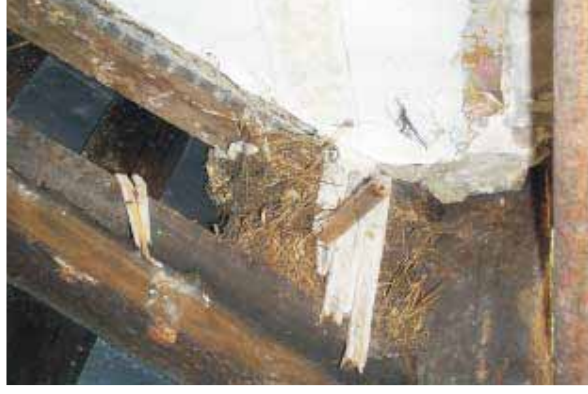
Plate 10: Eastern first floor room - insulation
