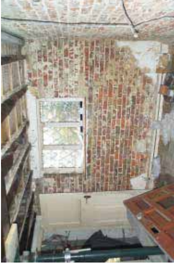
Plate 5: Western ground floor room - south wall
