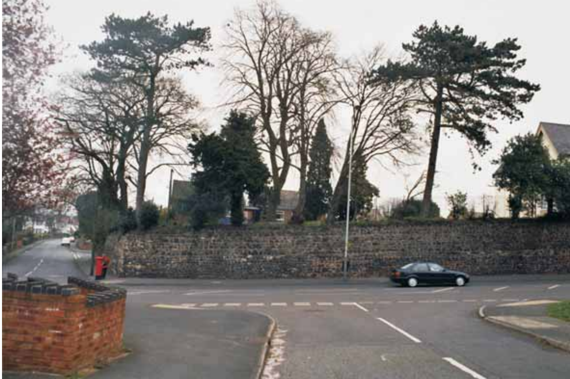
Plate 30: Clinker built retaining wall to Ivy Cliff [30]
