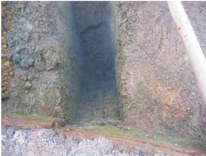
Plate 2: Geotechnical Survey Pit 2, taken from north
