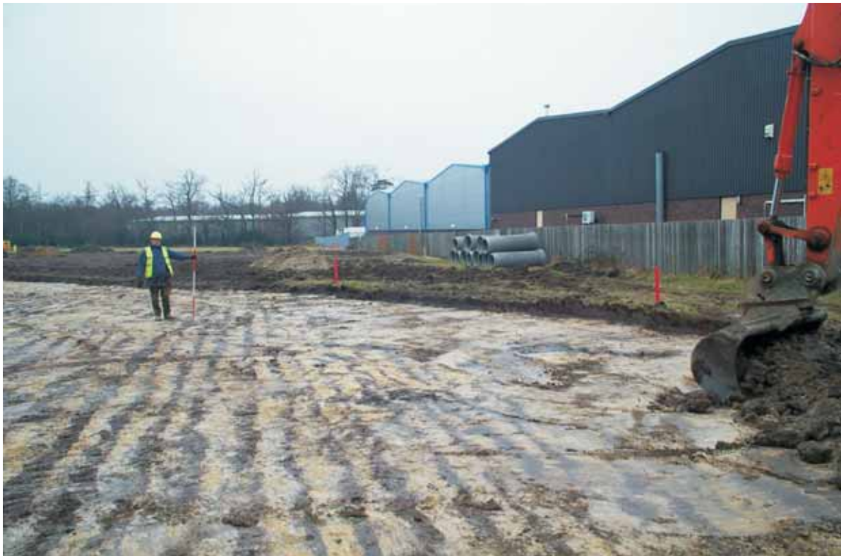
Plate 2: View from southeast of plough scars within the Access Road area
