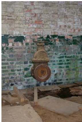
Water cooling valve
