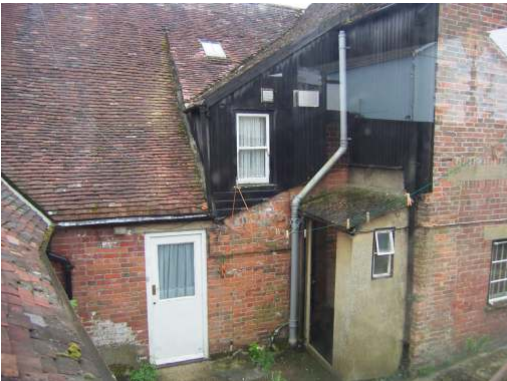
Plate 11: Rear of main building showing extensions and entrance to stairs
