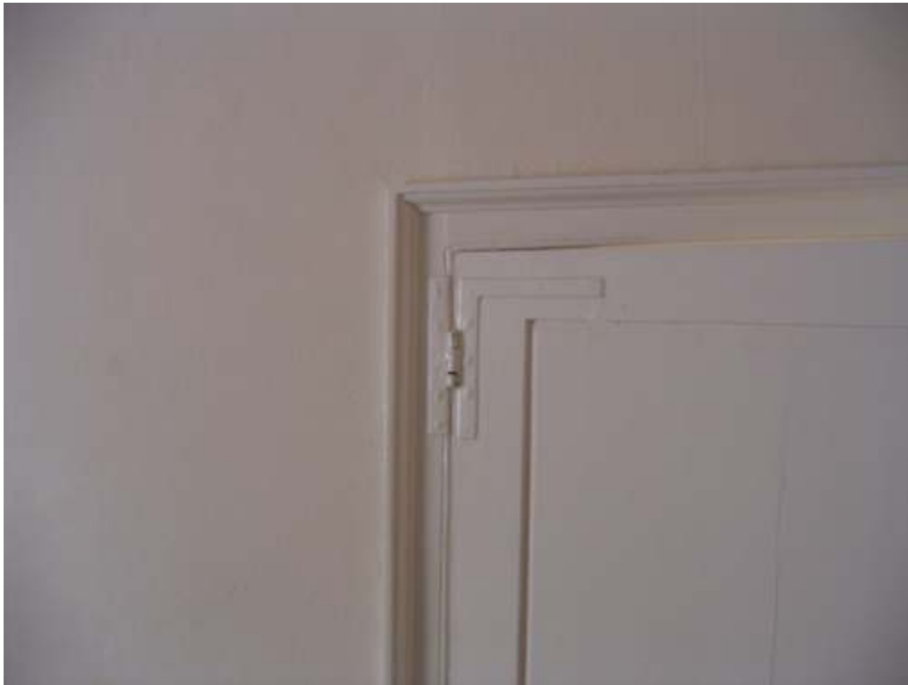
Plate 4: Detail showing early 18th century 'L' hinge on first floor door
