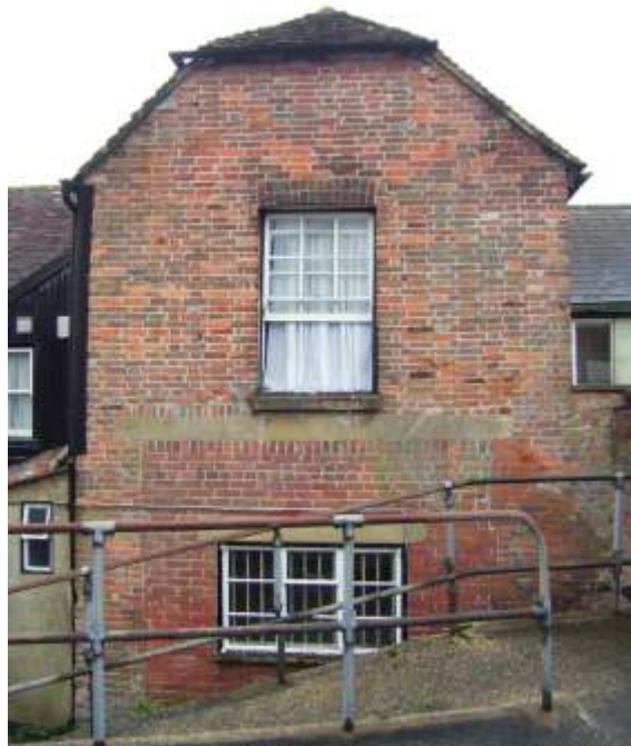
Plate 5: North west wall of two storey wing
