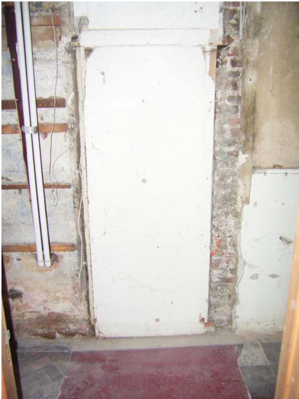
Plate 3: Blocked 18th century doorway
