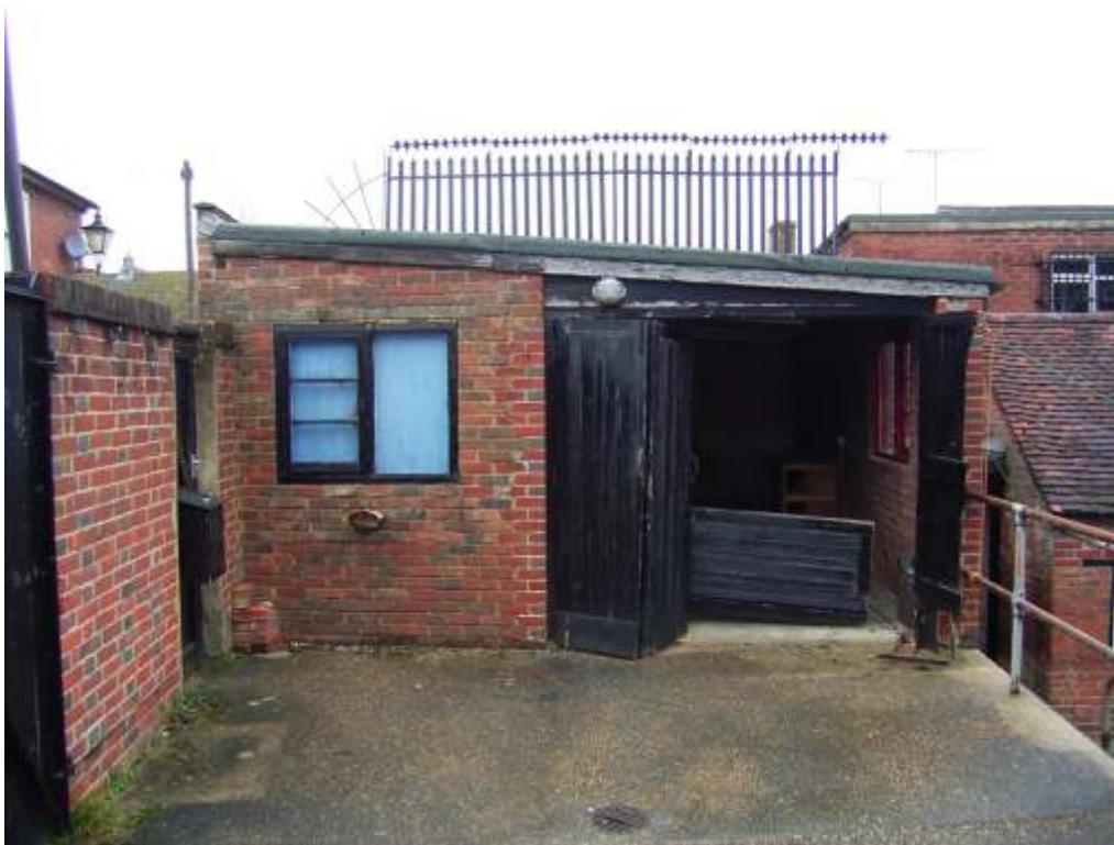
Plate 13: South west wall of garage
