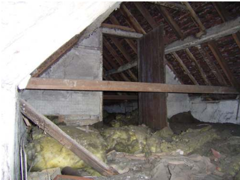
Plate 9: Present attic space
