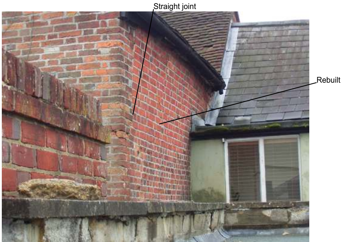
Plate 6: South west wall of two storey wing
