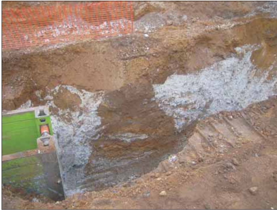
Plate 1: Swallow hole beneath quarry pit 3105 viewed from the west
