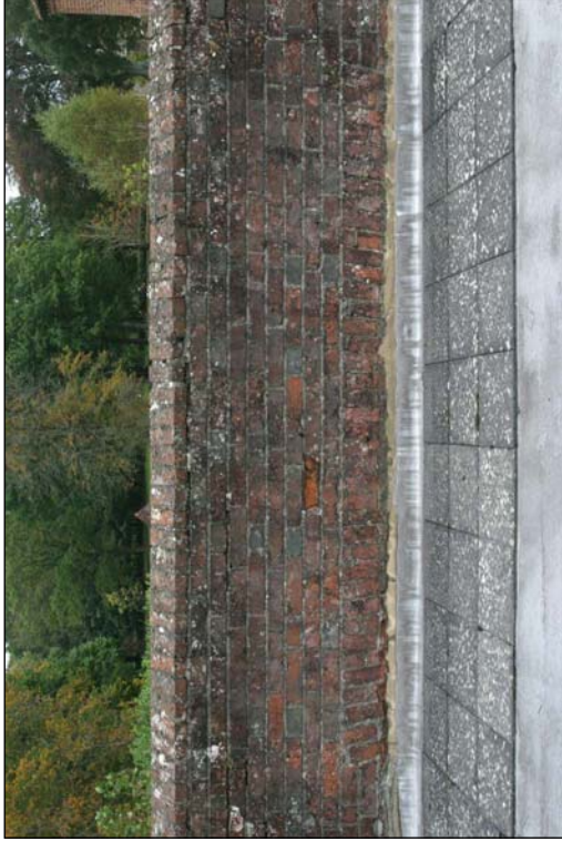
Plate A.1.3.p3: Flat brick arch of former opening in parapet above garages, looking north-east.
