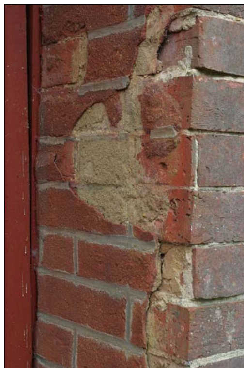
Plate A.1.5.p3: Detail of repair following creation of garage openings.
