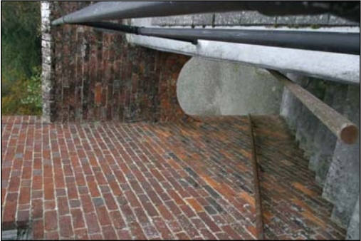
Plate A.1.4.p2: Brickwork of south-east wall of coach house showing change in build.
