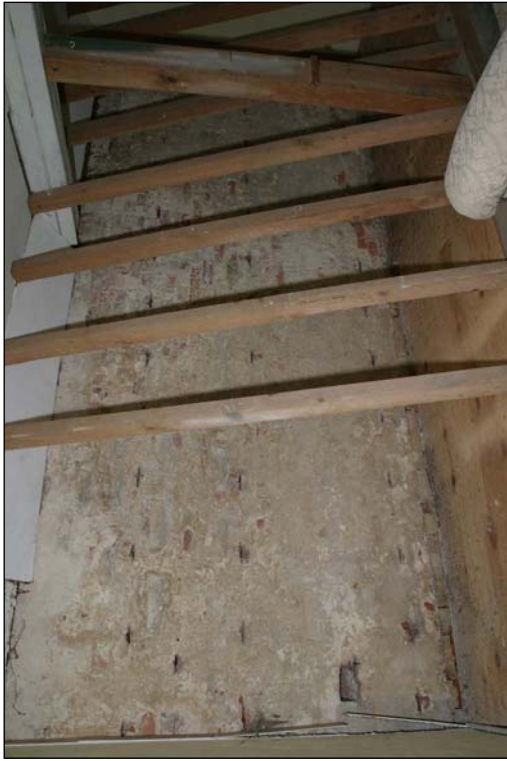
Plate A.1.2.p7: Internal propping in east room at first floor.
