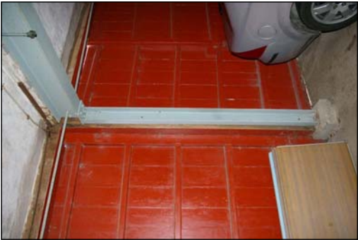
Plate A.1.2.p3: Interior of coach house doors showing supplementary steel structure.
