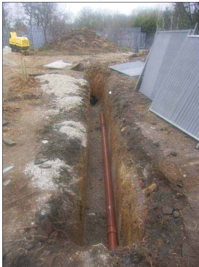
Plate 2: Pipe trench from northeast
