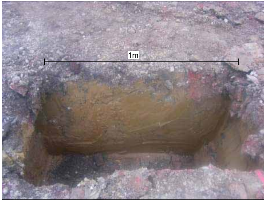
Plate 1: Building footing trench from southeast
