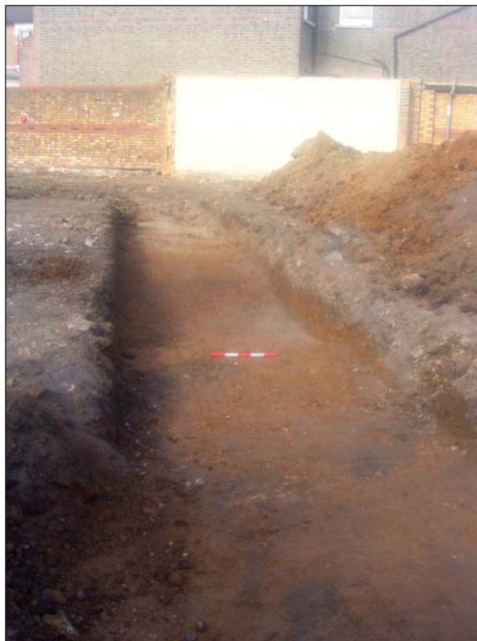
Plate 2: Trench from south
