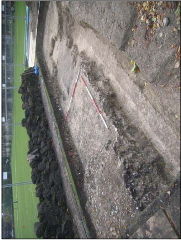
Plate 5: Wall 206 from north showing broken keying-in stones 251 and base mortar spread 261
