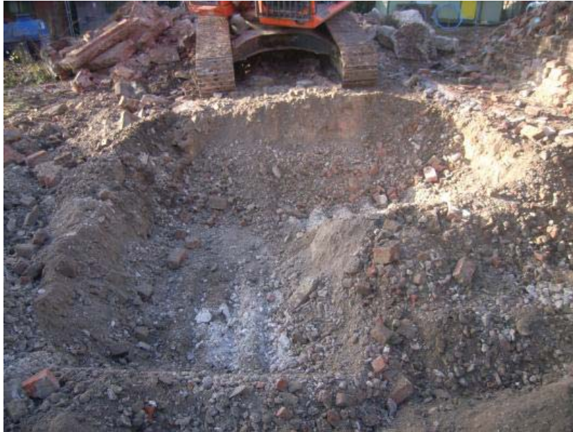
Plate 1: View looking north of exposed natural chalk underlying made ground.
