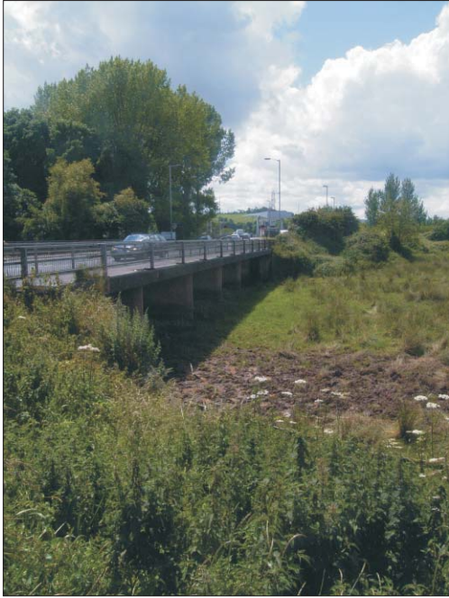
Plate 1: General view of site, viewed from the north-west
