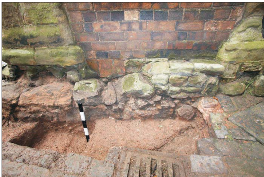
Plate 10: South facing section of Trench 1 showing foundation beneath 19th century blocked opening, later repair, and hanging tiles
