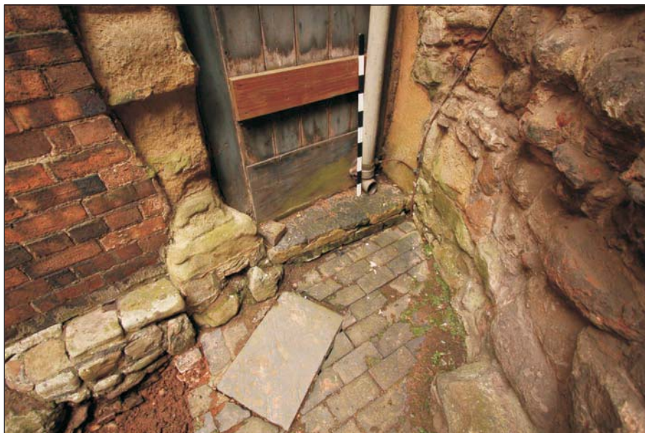
Plate 5: East blocked opening showing patterned tile step
