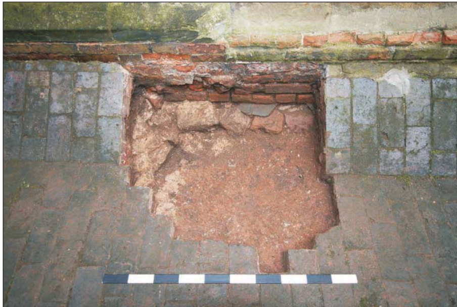
Plate 11: Trench 2 showing foundation for bay window (splay to left). 16th century walling to right of image, 18th century walling to left
