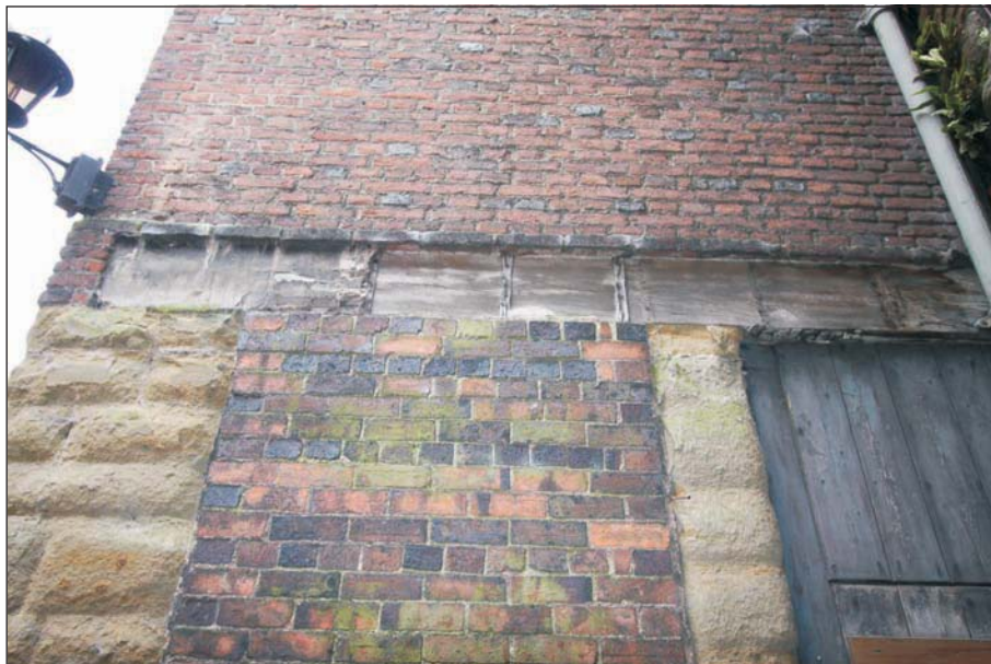
Plate 3: Horizontal beam spanning between piers
