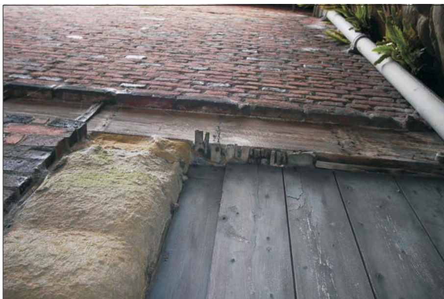
Plate 4: Detail of remnant lath and plaster on soffit of beam
