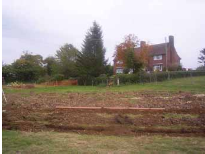
Plate 1: Irrigation trenches under excavation
