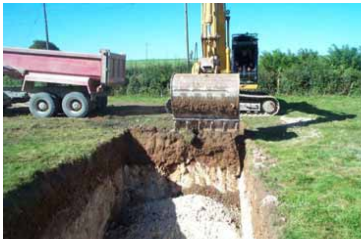
Plate 3: Excavation of settling tank trench
