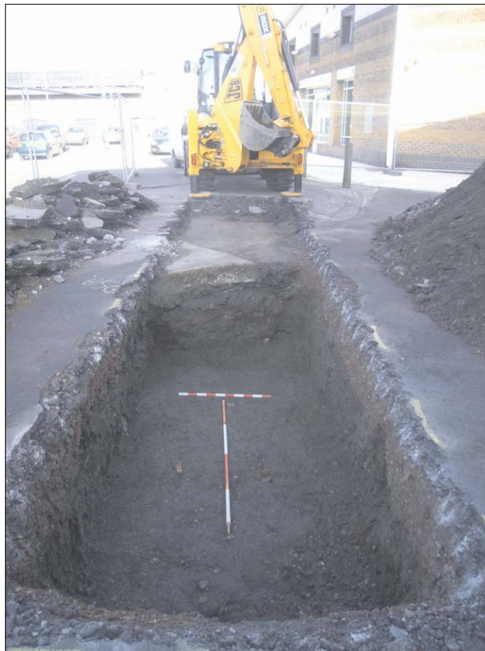
Plate 4: Trench 4 from south
