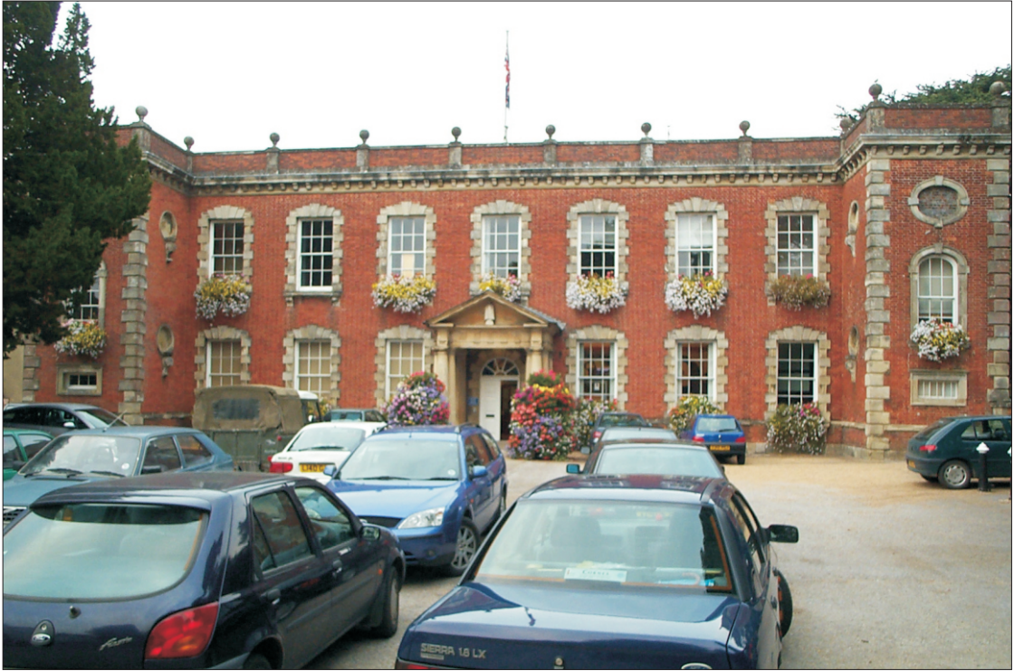
Plate 1: Rear view of Bournehill Council Offices (Area A) taken from the south
