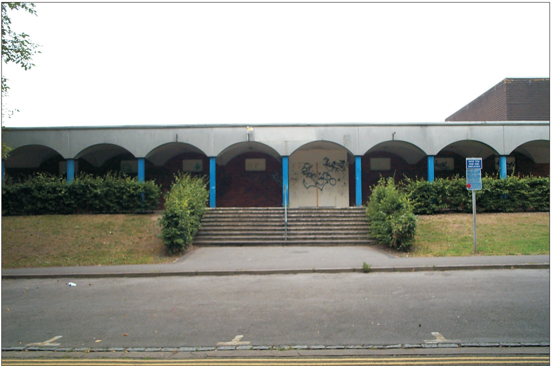
Plate 2: Swimming Pool (Area B) taken from the south
