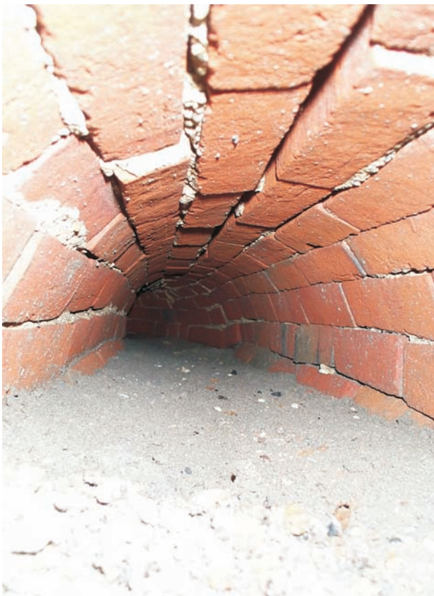
Plate 3: Interior of drain 215, looking west
