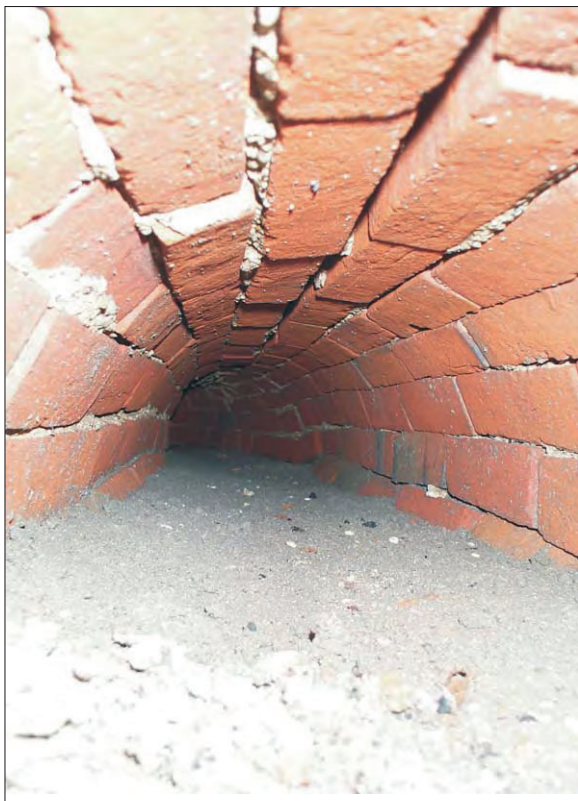
Plate 3: Trench 2 - Interior of drain 215 , looking west
