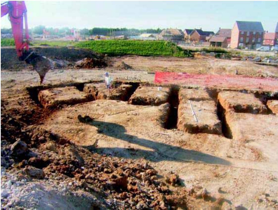
Plate 3. Phase 3 - Footing excavations
