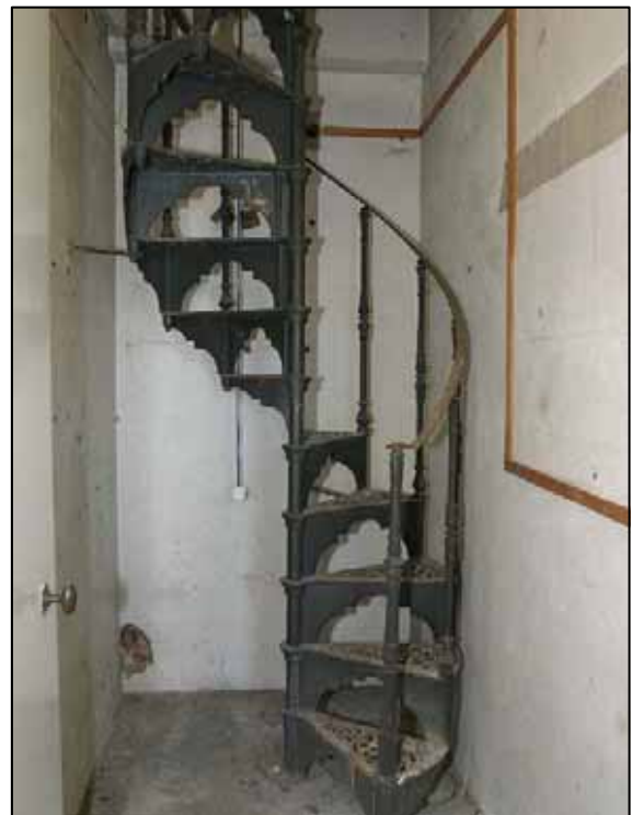
Plate 6: Access to clock tower via spiral cast iron staircase
