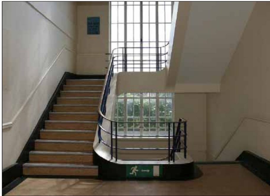
Plate 11: Building A: Staircase with cast iron balustrade and brass handrail
