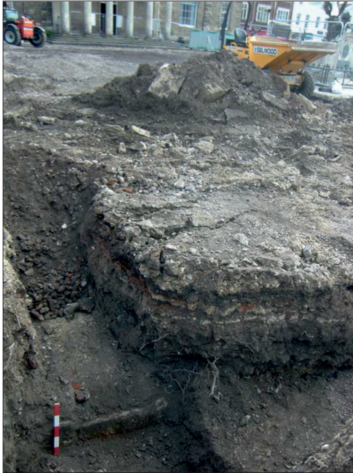
Plate 3: Structure 114 , exposed in base of pipe trench (view from north; scale = 0.5m)
