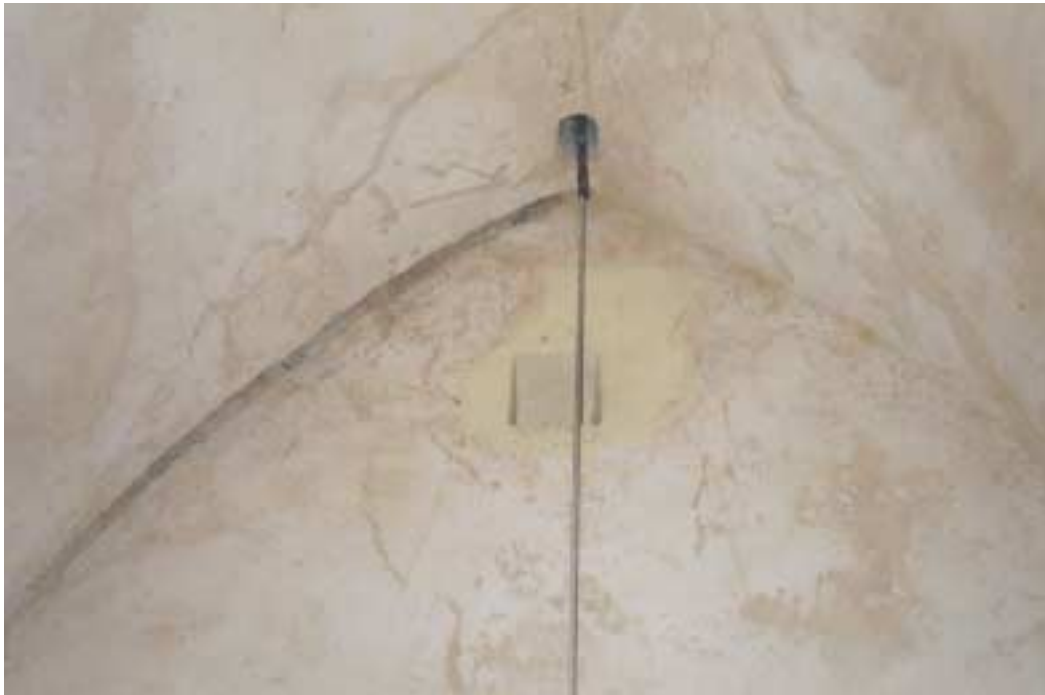
Water may be entering the chapel at the west end through the bell rope hole
