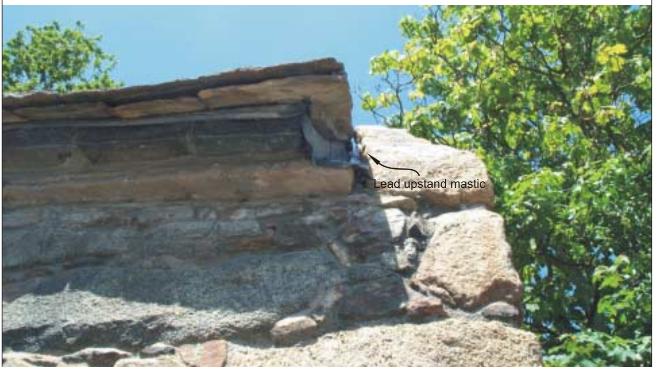
One of the lead-lined gutters a potential source of water ingress.
