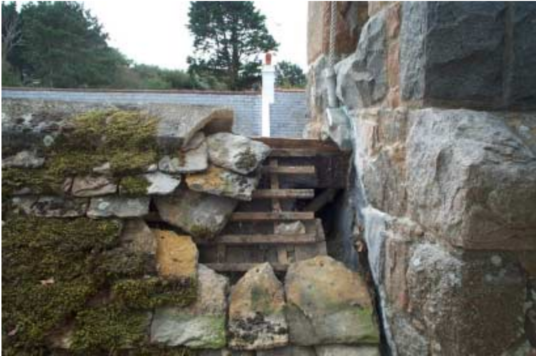
Area 3: removal of Cotswold stone roof slates.
