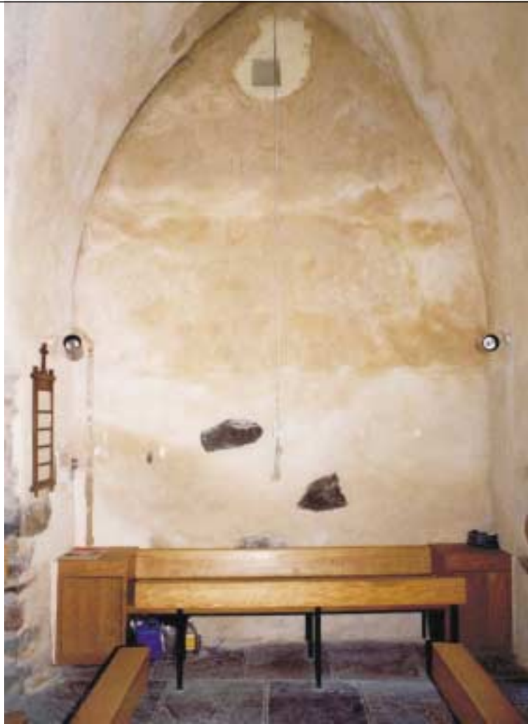
The west wall is badly stained by water ingress
