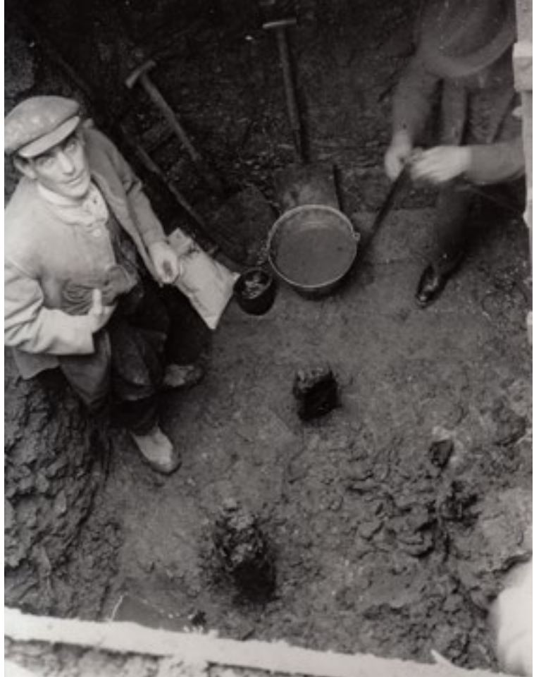
Minimal trench shoring and no protective clothing on an excavation c.1927-1930 © Museums Sheffield
