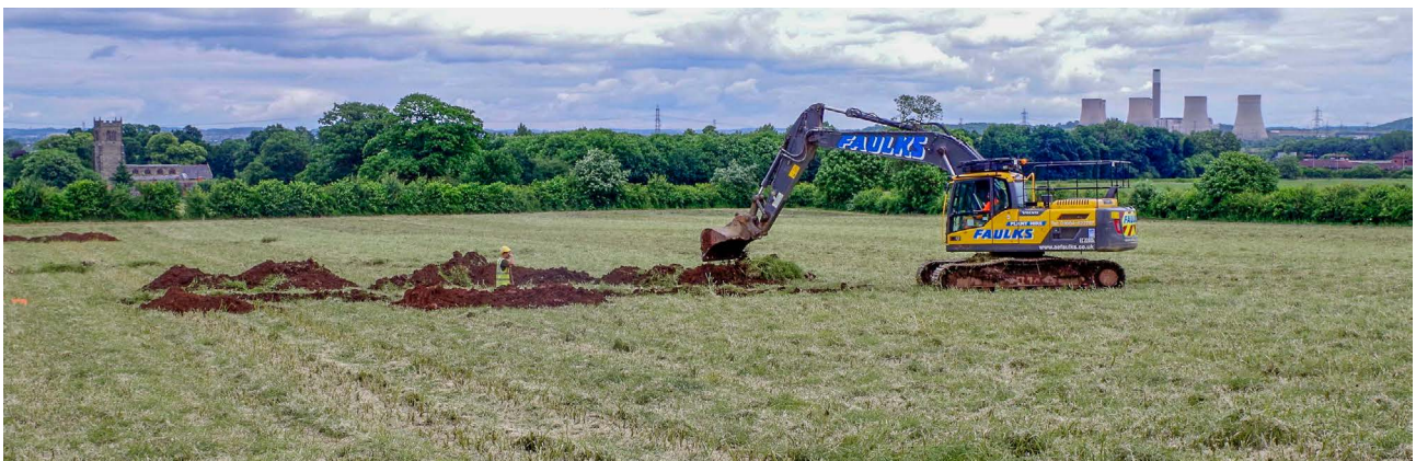
Plate 1.2 Evaluation: Michael Keech monitoring trenching near Lockington
